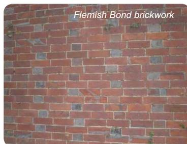
Flemish Bond brickwork
